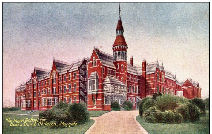
This view shows the 1875 school building. The image can be compared with Christopher Alexander's oil-painting above
